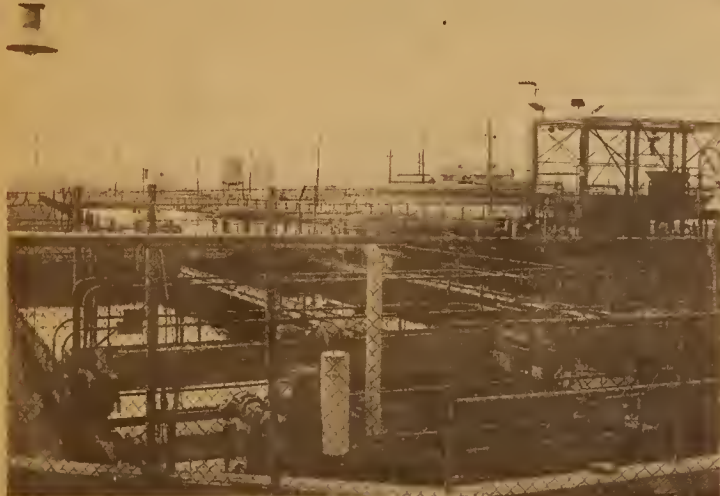
Waste Treatment Facility
