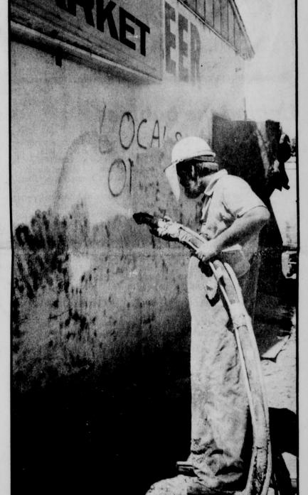
BLAST OFF — The graffiti slogan 'Locals Only' gets blasted off the wall of A&M Market, as Chuck Moore of Nor Cal Coating sandblasts the Healdsburg Avenue store in preparation for a new coat of stucco.
