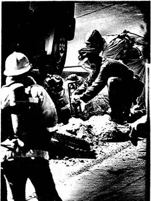
Handy in a Pinch—Gas company crew lowers contractor on Activity Road north of Black Mountain Road. Area was evacuated briefly.
