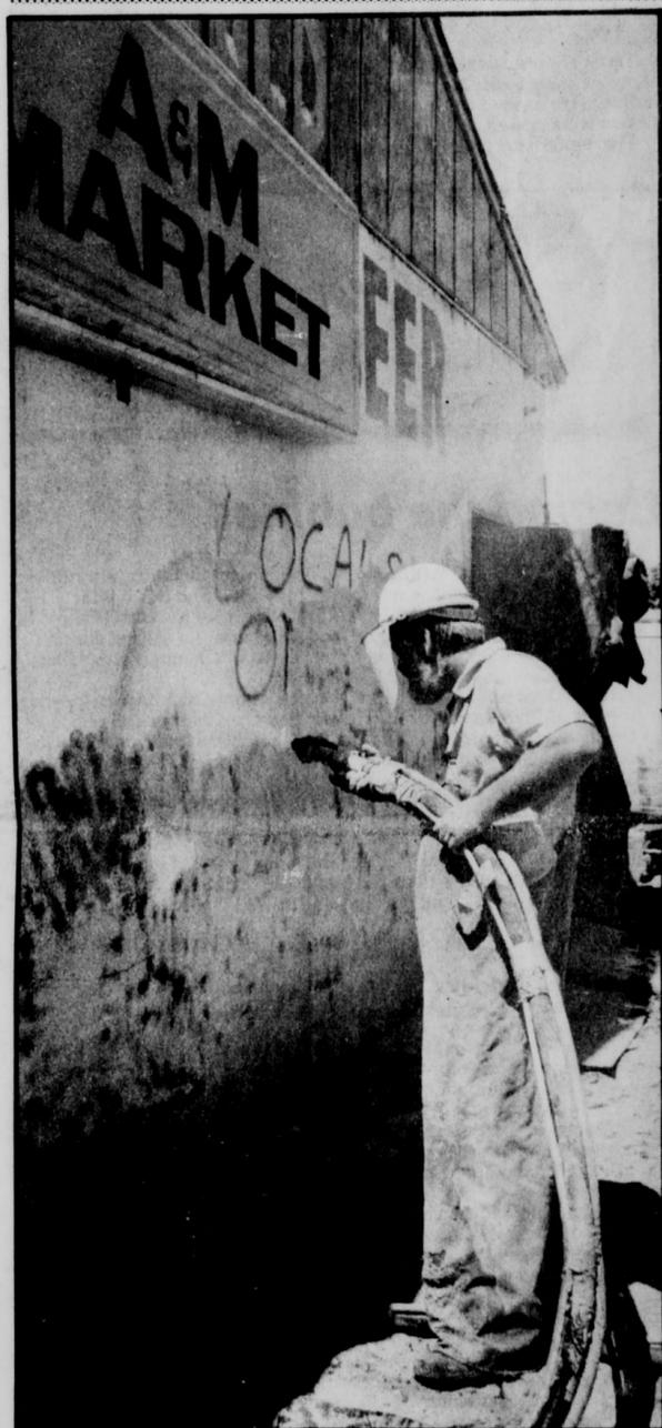
**BLAST OFF** — The graffiti slogan 'Locals Only' gets blasted off the wall of A&M Market, as Chuck Moore of Nor Cal Coating sandblasts the Healdsburg Avenue store in preparation for a new coat of stucco.
